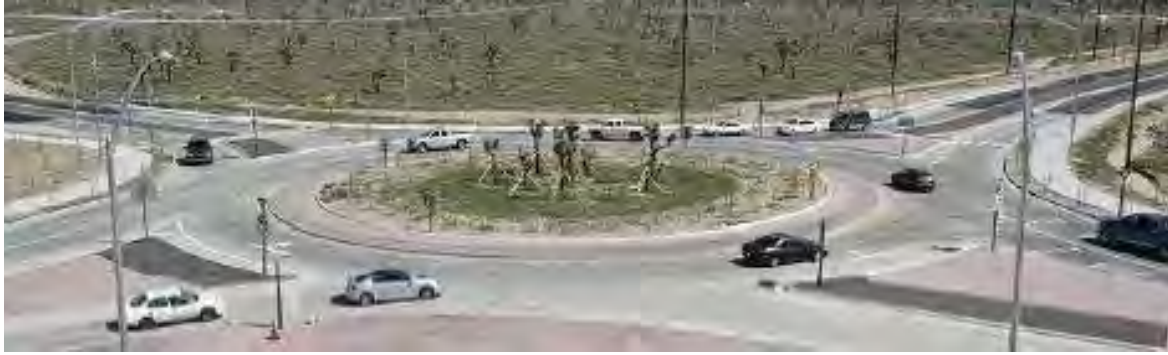
Roundabout on Route 138 in Palmdale
